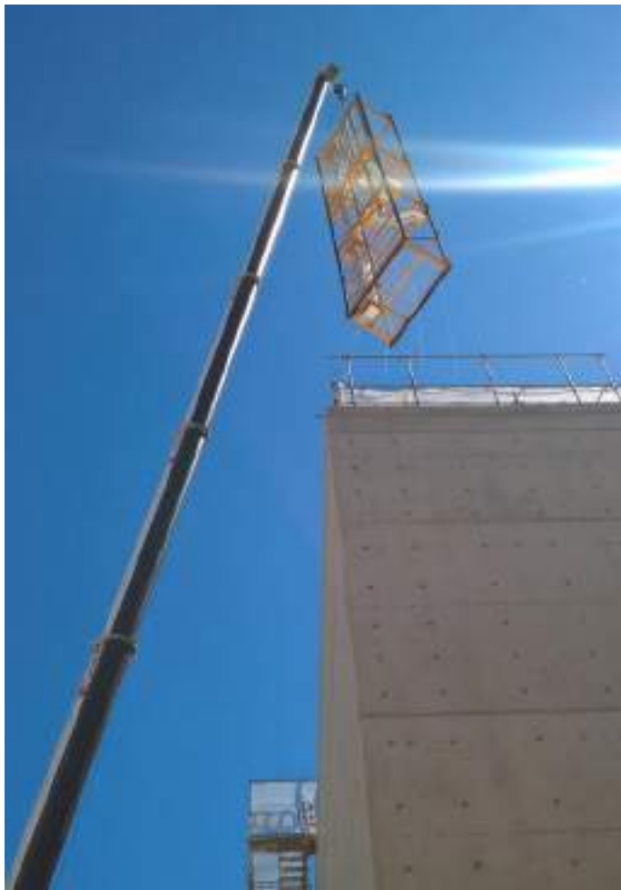
Figure 17 (Top): Hoisting of vertical riser module. (Photograph courtesy of Laing O'Rourke)
