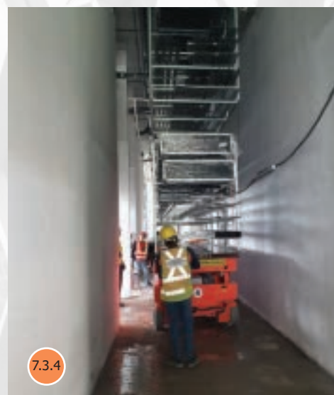
FIGURE 7.3.4 Lifting and installation of horizontal modules on site
