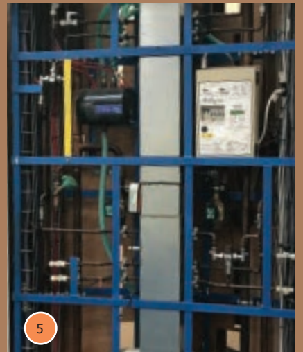
4. Prefab horizontal module with ceiling board | 5. Prefab vertical riser module with catwalk
